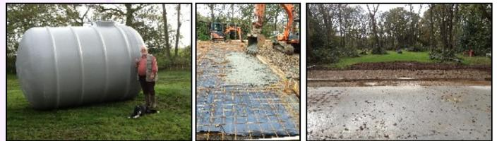
left to right ... Cesspool tank before being buried; Pouring concrete for the main foundation slab; Completed main slab - the verandah section about to be laid. [Click here](#) for more photos.
